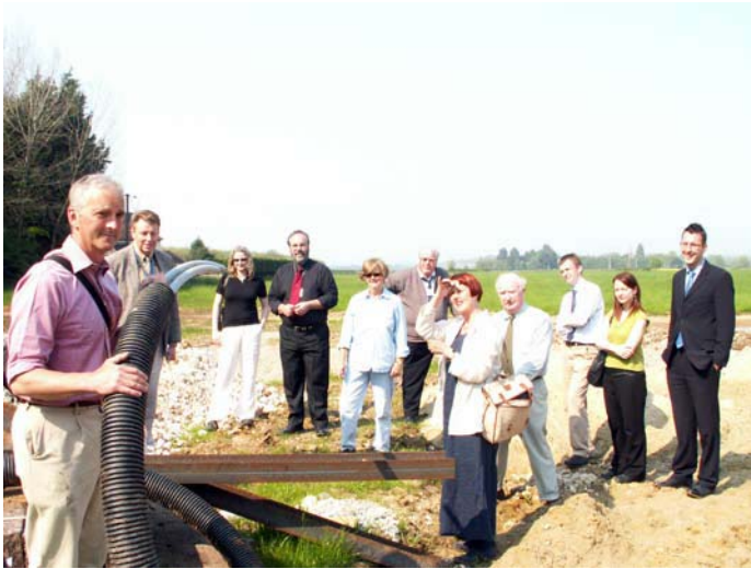
The group being shown insulated district heating network piping that will be used for transporting hot water from the biomass boiler to buildings, before it is installed underground.
