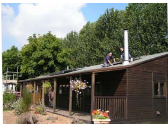
Solar technology being installed at Wildwood
