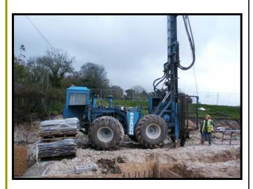
Only a few metres below the ground the temperature stays at around 11-12 degrees Celsius throughout the year. By using ground source heat pumps (GSHP), this heat can be sourced to provide space heating in the home, and in some cases help pre-heat water for the central heating system.
